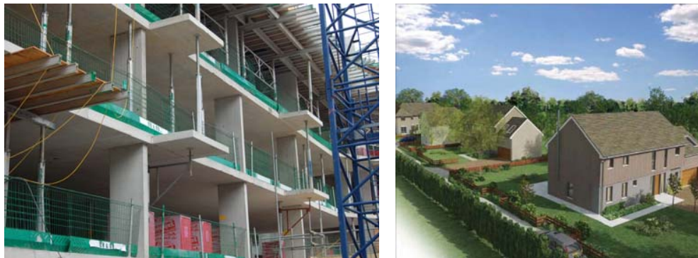
One Brighton, under construction (left), Springfields, Ifold, Artists Impression (right)
