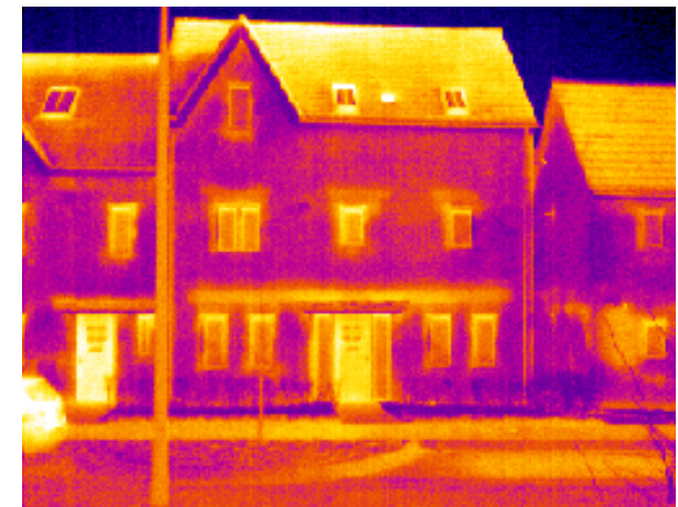
Stamford Brook, thermographic image
