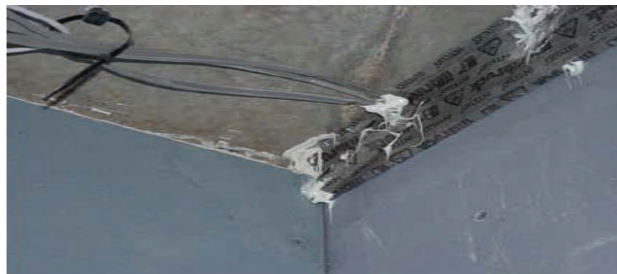
Leakage where membrane is poorly sealed around cables—use of grommets was recommended
