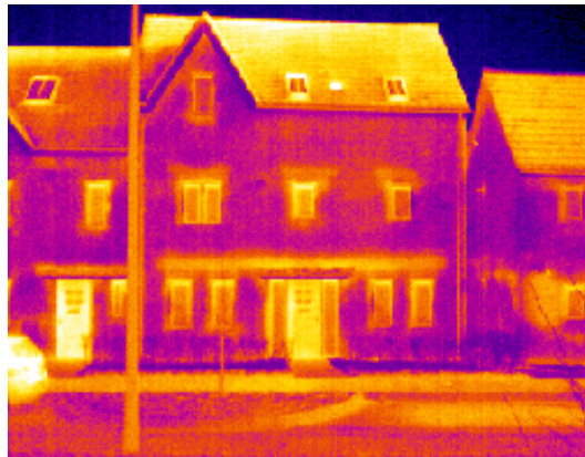
Stamford Brook, thermographic image:
